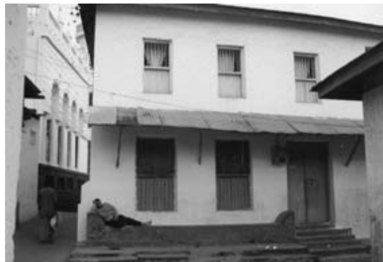
Figure 16 An Omani house in Old Malindi with built-in bench.
