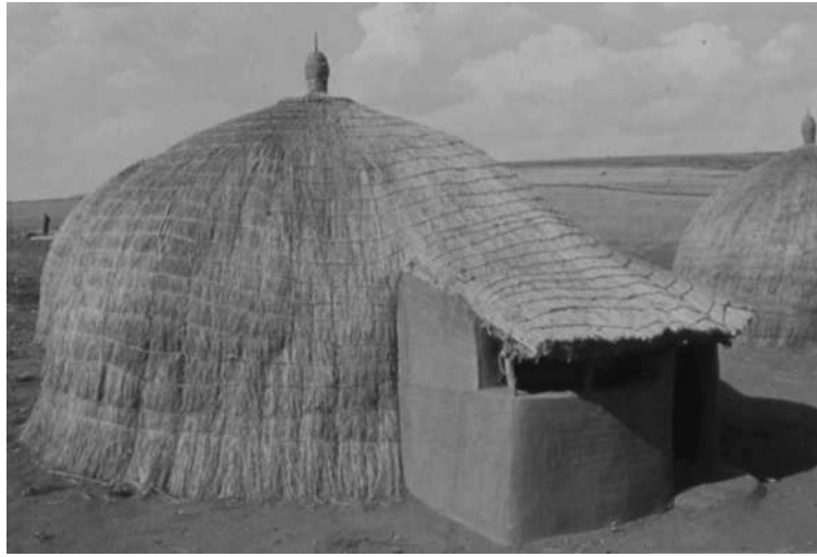
Figure 3 Verandah type doorway (photograph by the author).
