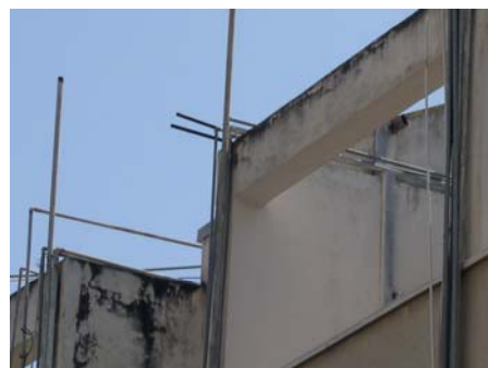
Figure 10: Fungal growth on a painted surface.
