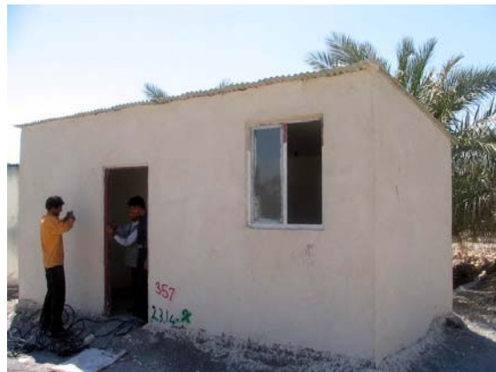
Figure 6: steel structure prefabricated houses with brick walls(18 m 2 )
