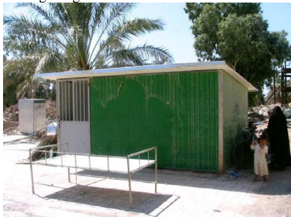
Figure 5: prefabricated temporary housing made with fiberglass(18 m 2 )
