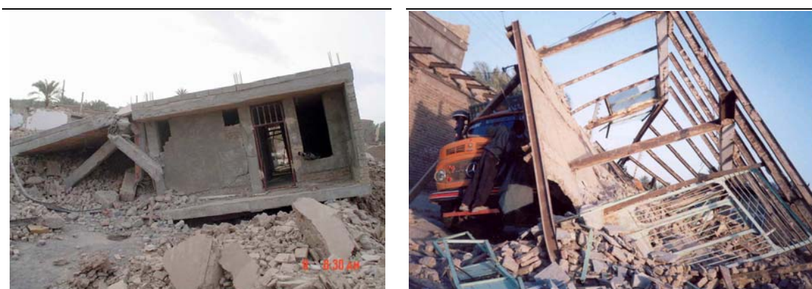
Figure 2: Destruction of concrete and steel structure buildings near earthquake epicenter due to incorrect erection
