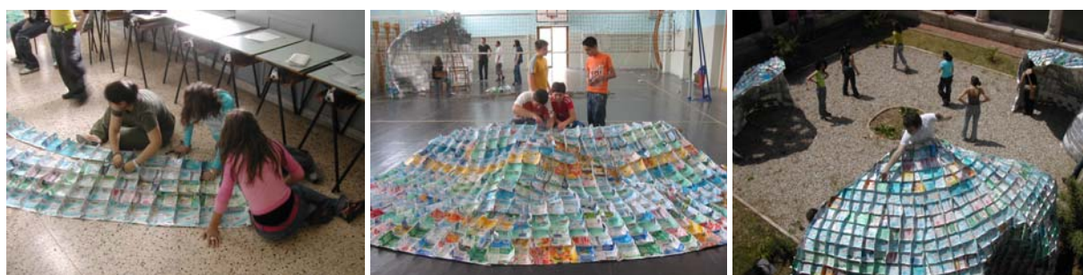
Figure 3,4 & 5: assembly steps of cardboard lightweight shells
