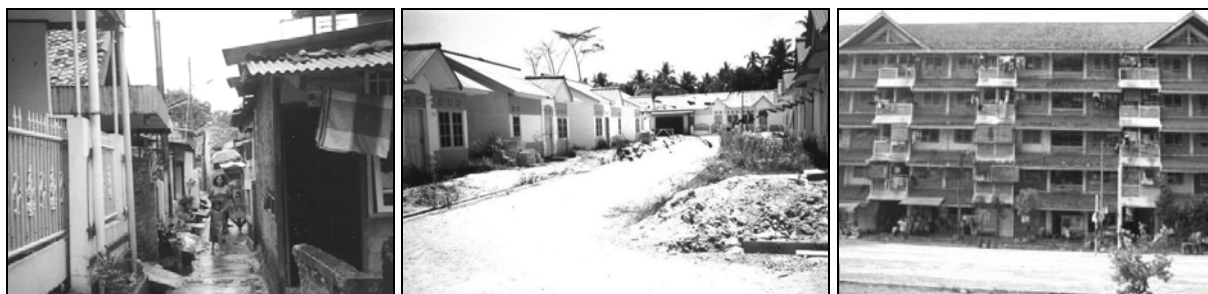
Figure 1: Typical street-level situation in Kampung (left) compared to resettlement housing in Rumah-sederhana (middle) or Rumah-susun (right)
