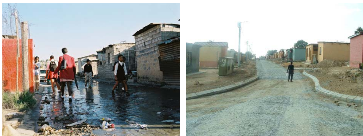
Figure 7: Improving infrastructure such as roads
