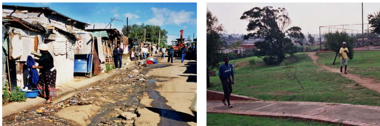
Figure 8: Improving infrastructure to make it more pedestrian friendly
