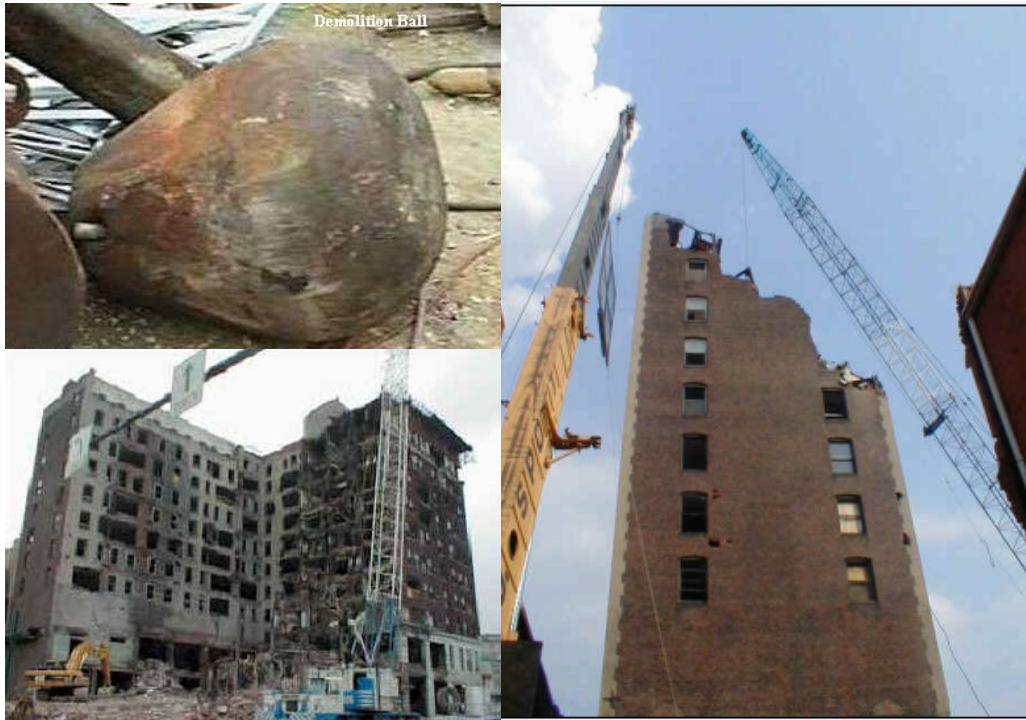
Figure 7: Deconstruction Examples by Steel Ball [7], [8].
