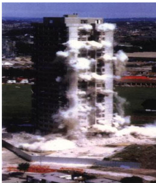
Figure 8: Deconstruction of a High Building by Explosives [9].
