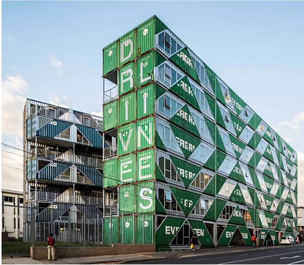
Figure 2. Street view of the container building comprising businesses and residences. (Photo credit: Driveline Studios).
