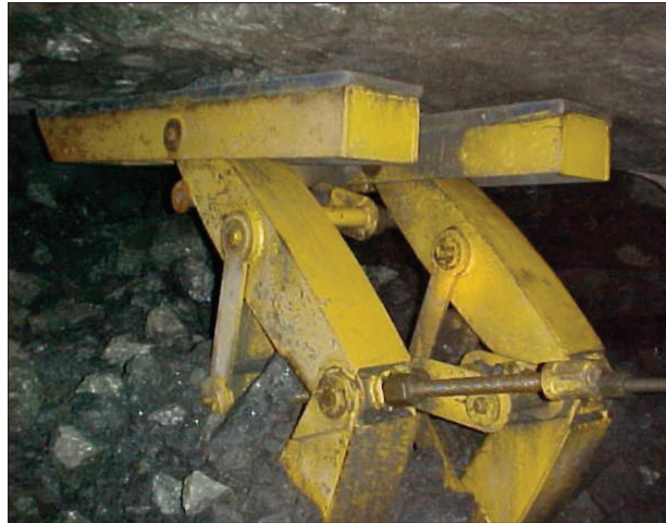
Figure 10—The original version installed underground after blast. Note the threaded rod sticking out the back
