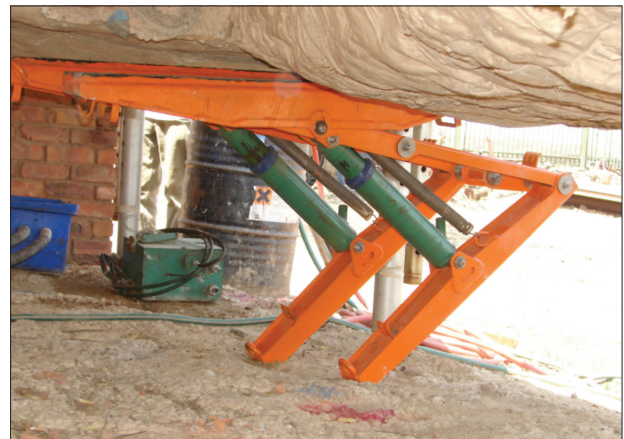
Figure 9—A preproduction unit undergoing trials in the stope. Note the prestress device pump in the background
