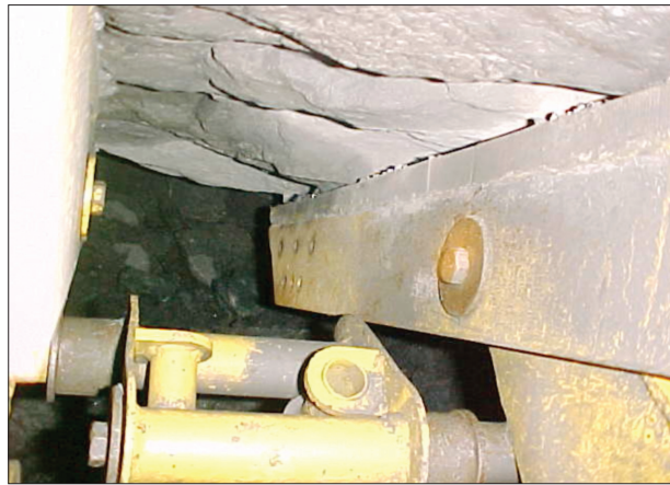
Figure 11—Photo of roof support system supporting loose rock after a blast
