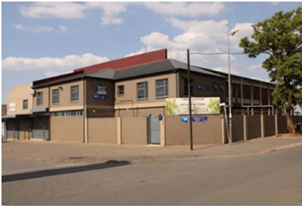
Figure 5. The Tshwane Play House after refurbishment (Source: Author).
