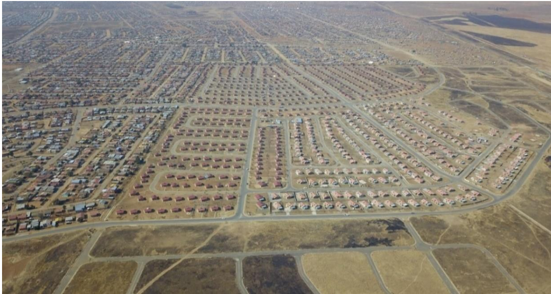
Figure 4.2: Hillside View (post construction, October 2021)
