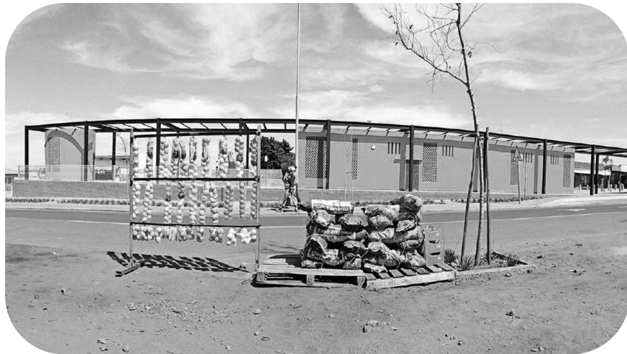
Figure 4.10: Illustrating the isolation of the Refilwe Business Node with the community. The community does not interact with the structure as intended by the designers. This photograph shows the alienation of the business node (Feat 2014).
