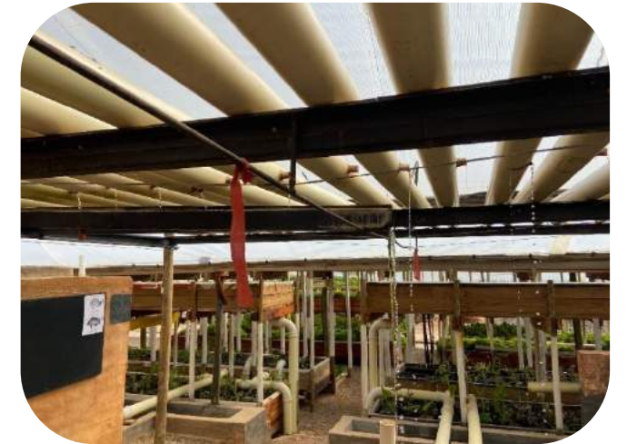
Figure 5.25-5.26: Illustrates the natural fall of pumped water breaking the surface of the water which is the only way oxygen is achieved in the fish tanks. Photo by Author 2021 (Author 2021).
