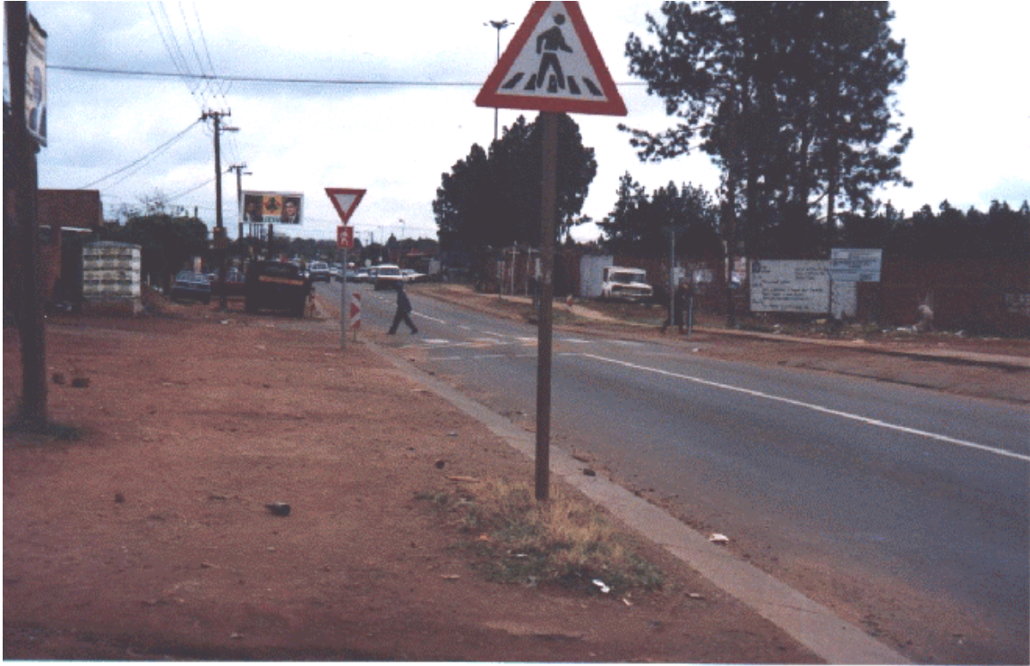
Photo 1: Pedestrian Crossing. Note unpaved sidewalks
