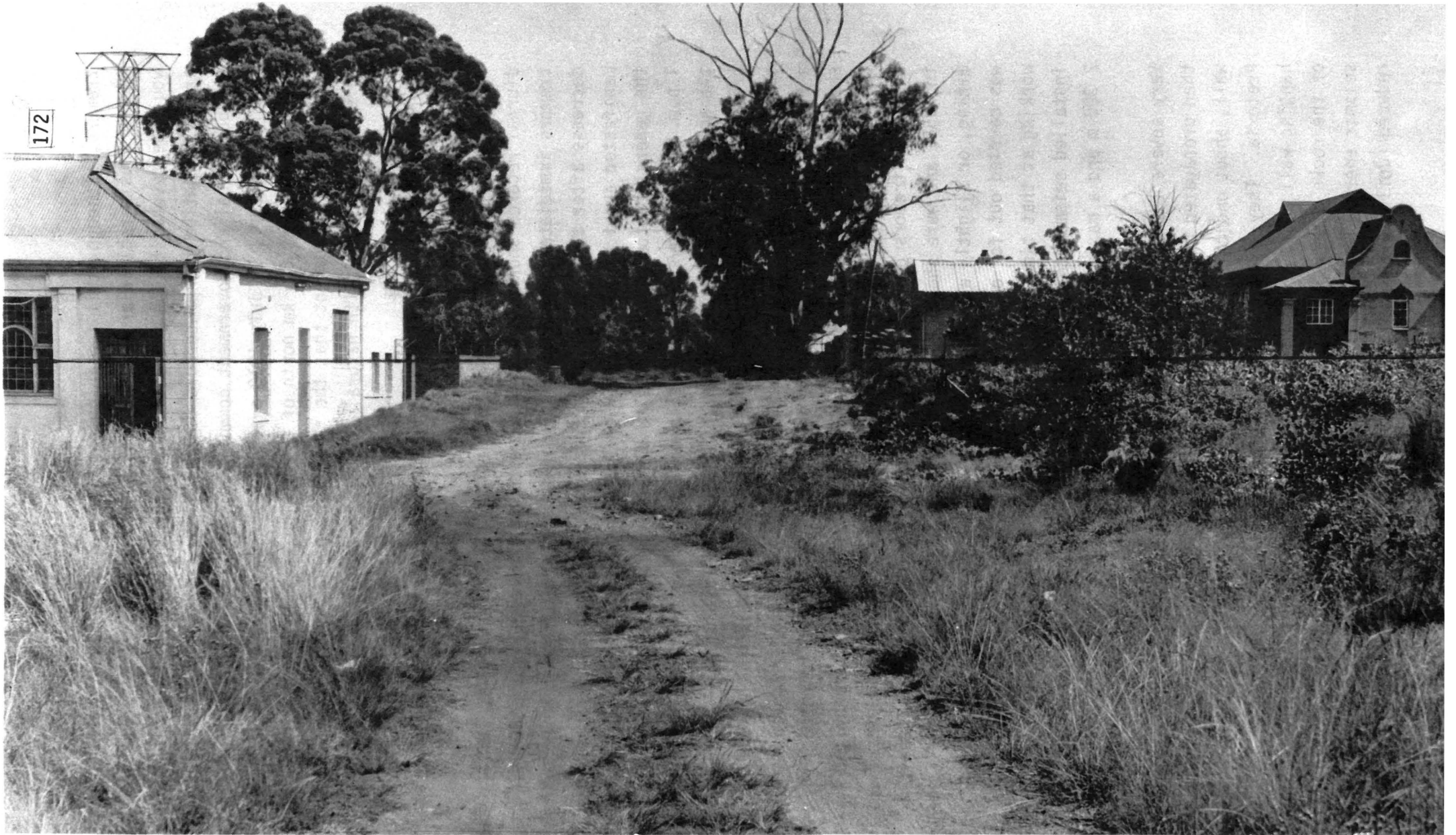
FIGURE 5/43 : Two old mine houses in Cleveland, Johannesburg : house 'A' on the right is situated on the dyke while house 'B' on the left is just off the dyke, the dyke running behind the house ; the amount of subsidence can be judged by the difference in ground level between the two houses, house 'A' being situated at original ground level as indicated by horizontal line.
