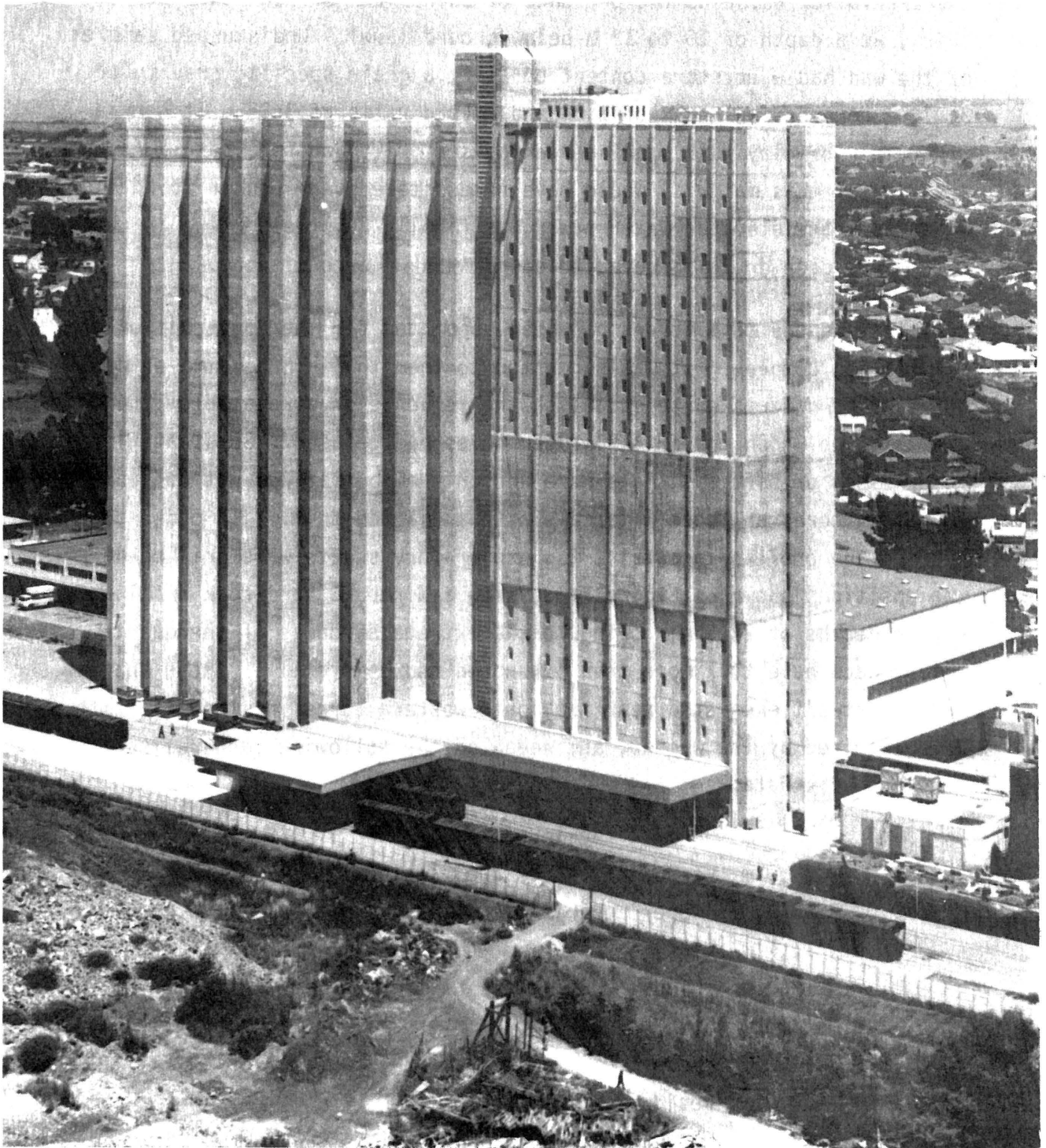
FIGURE 7/37 : Mill and silo complex, Randfontein : the tallest silos in Africa.
