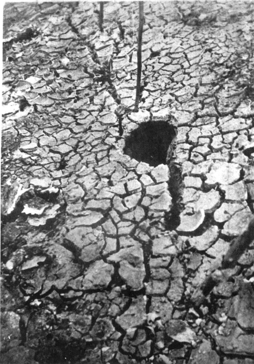
FIGURE 3/20 : Small 'sinkhole' in floor of Westphalia Leidam
