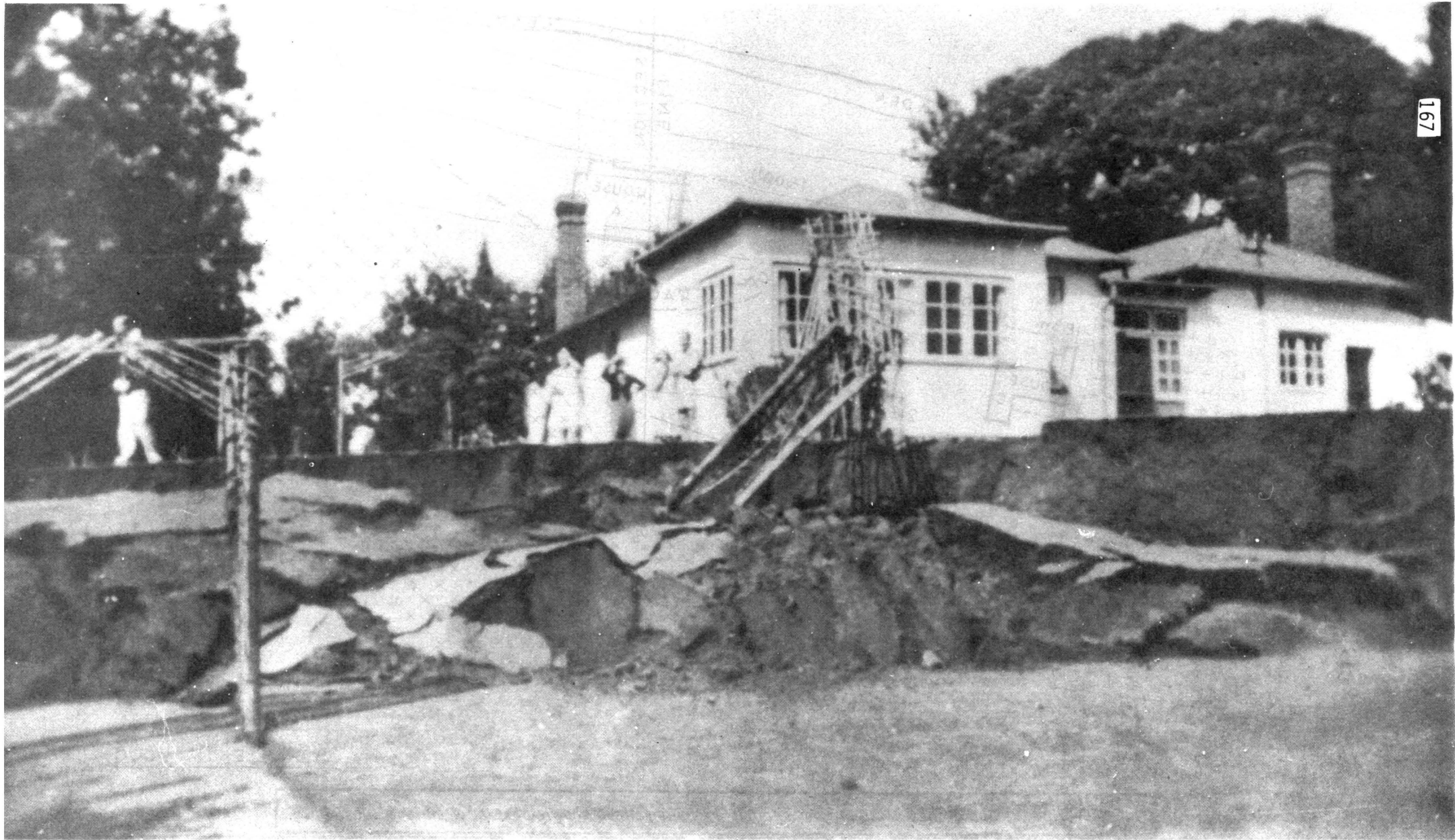
FIGURE 5/39 : 'House B' at Nourse Mines photographed from the north after the subsidence of 3rd May 1942 showing the line of fracture
