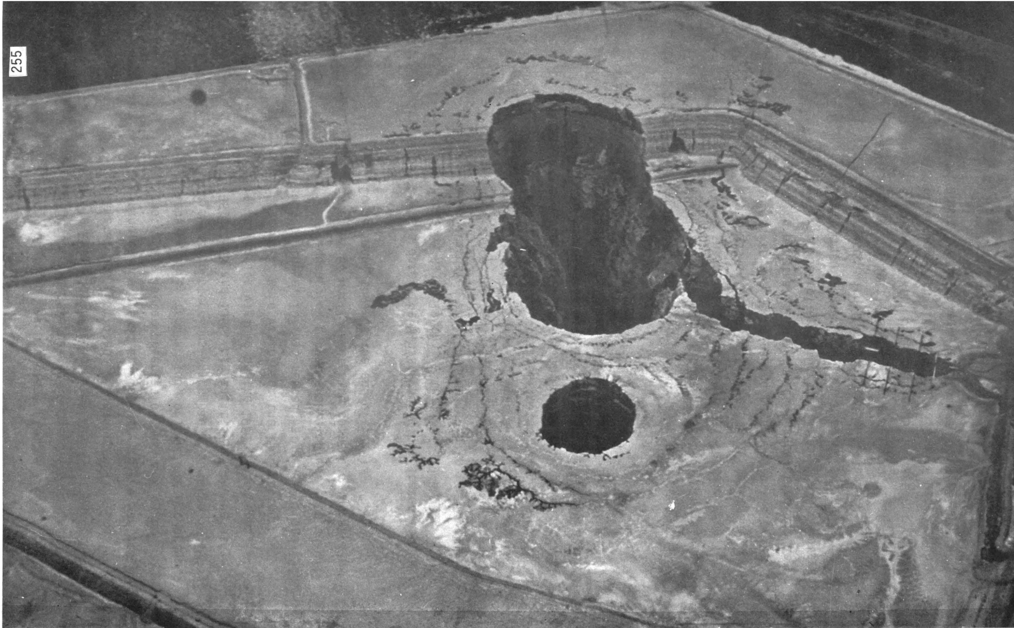
FIGURE 7/25 : Sinkhole at West Driefontein slimes dam
