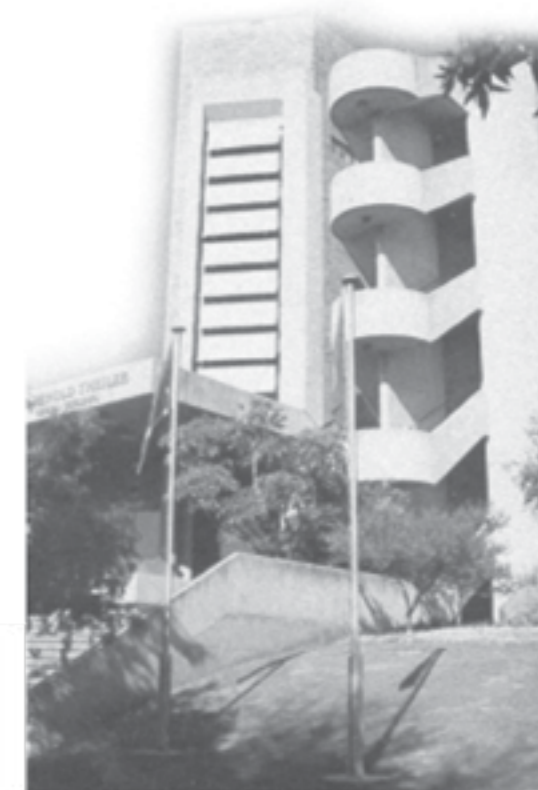
Arnold Theiler Building
