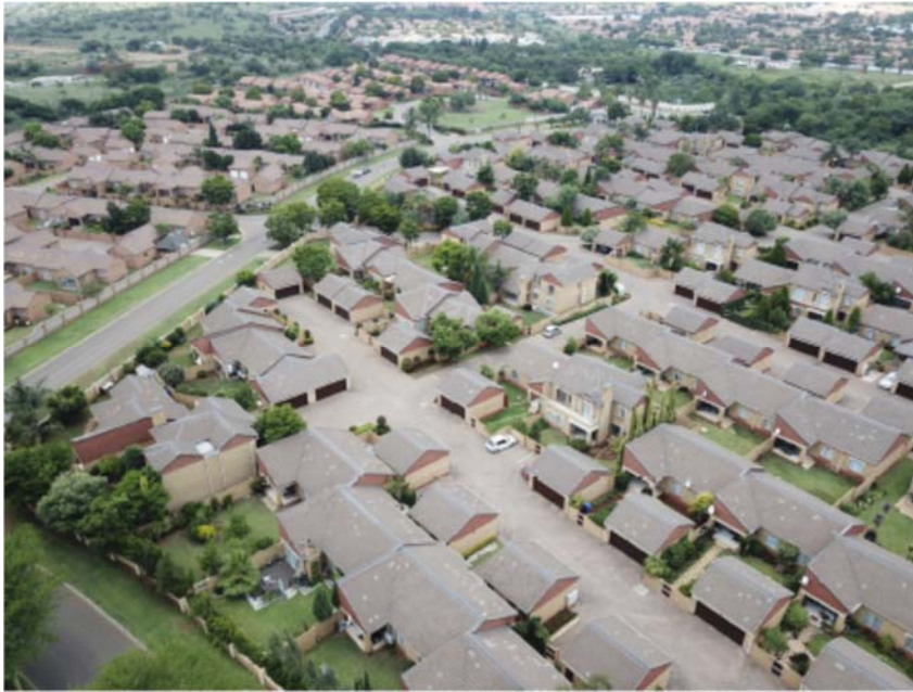
Plate 2. (Aerial view of Equestria Estate)
