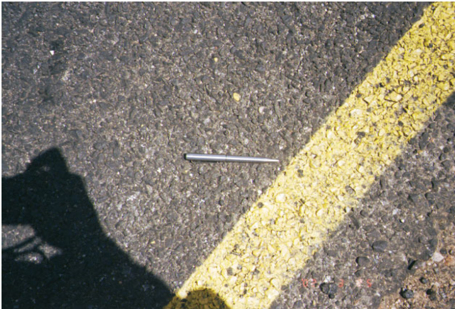
Figure 10: Close up view of the seal after one year
