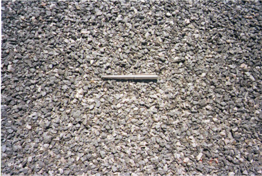
Figure 9: Close-up view of the second layer on top of the first layer before application of the fog-spray
