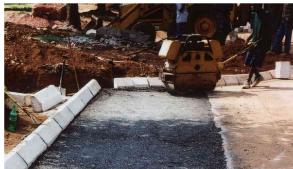
Figure 6. Compaction of FTBC
