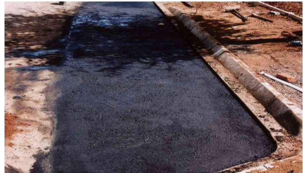
Figure 9. Completed test section
