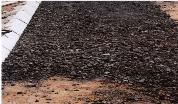
Figure 6. Segregation of FTBC mix
