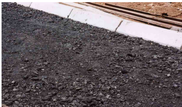
Figure 5. FTBC prior to compaction
