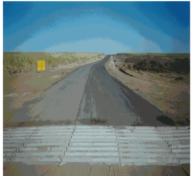
D 348 Mount Elias – After upgrading to low volume surfaced standard.
