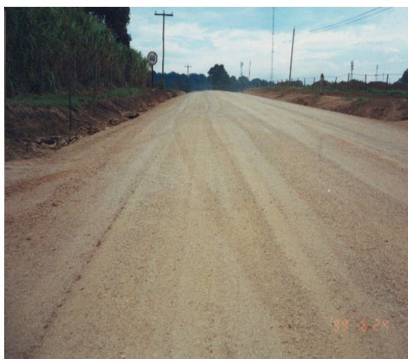
D425 Alverston – Waterproof Gravel just after construction
