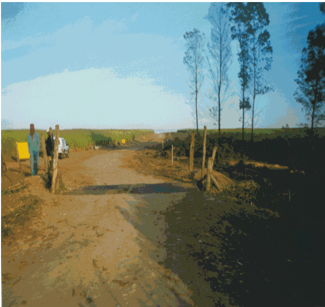
D 348 Mount Elias – Before upgrading to low volume surfaced standard.
