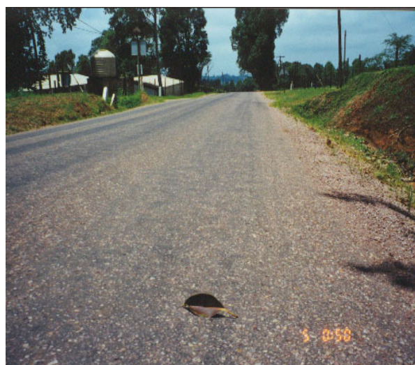
D425 Alverston – Waterproof Gravel 8 months after construction
