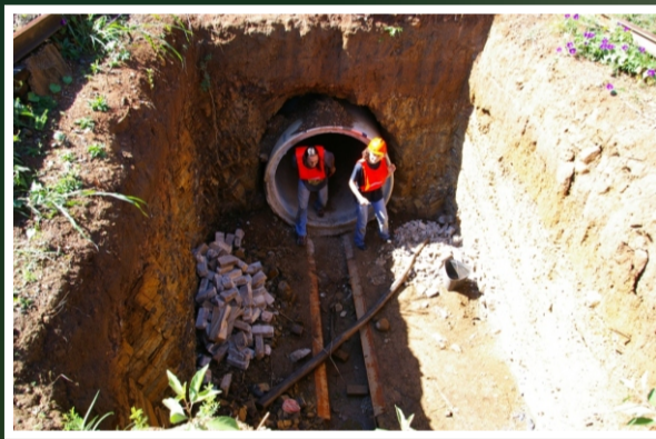
Figure 3: Entrance to the 1.2 m high tunnel (depth = 38.8 m)
