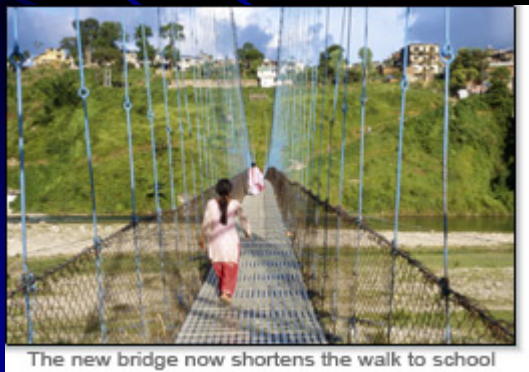
The new bridge now shortens the walk to school
