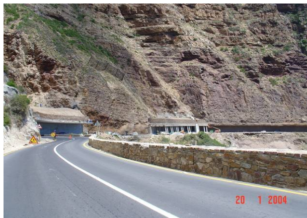
Photo of Road Showing Cantilever Canopy Propped Canopy and Half Tunnel
