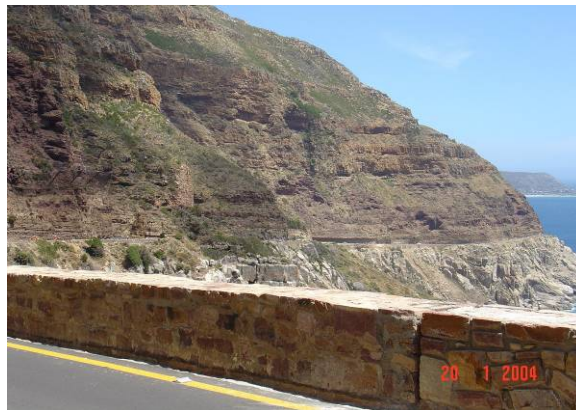
Stone Packed Retaining Walls
