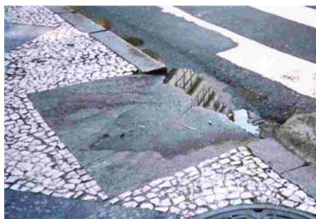
Figure 5: Kerb ramp not aligned with the street. Photo: SHTV/2004
