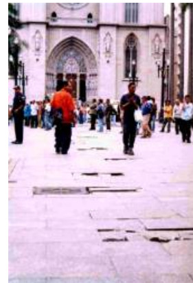
Figure 4: Sé square, loose granite slabs. Photo: SHTV/2004
