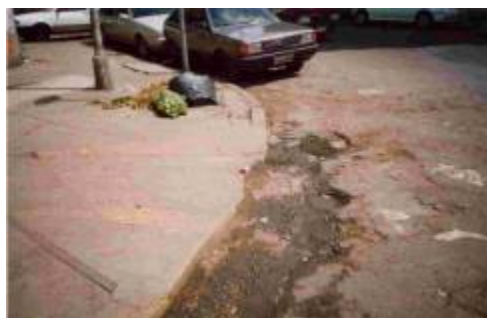
Figure 6: Kerb ramp according to the norms, but the street surface is full of holes. Photo: SHTV/2004
