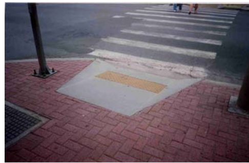
Figure 13: João Cachoeira Street. Pilot project with pre-molded kerb ramps. Picture: SHTV/2005
