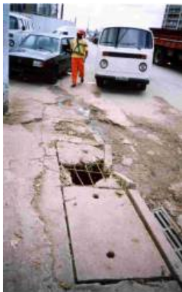
Figure 3: Gutter in poor state. Photo: SHTV/2004
