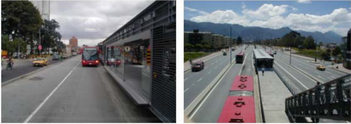
Figure 9. Example of bus road and station.
