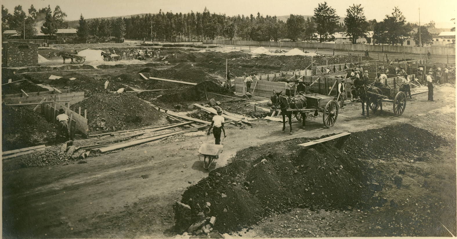
• Commencement of Work • • Excavation & Foundations •
