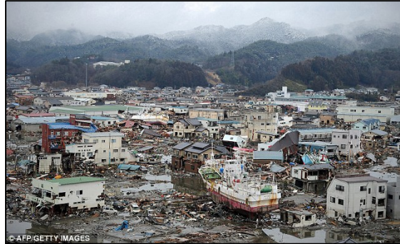
b) Damage caused by the tsunami on 11 March 2011 in Kesenuma, Japan (Photo: http://www.dailymail.co.uk )
