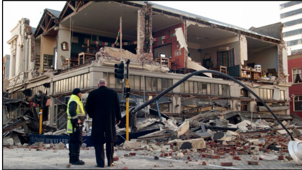
a) Damage caused by the earthquake on 4 September 2010 in Christchurch, New Zealand (Photo: www.foxnews.com )
