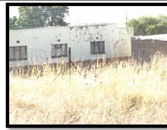
Photograph 3.12: Typical houses in the community, 29 May 2014
