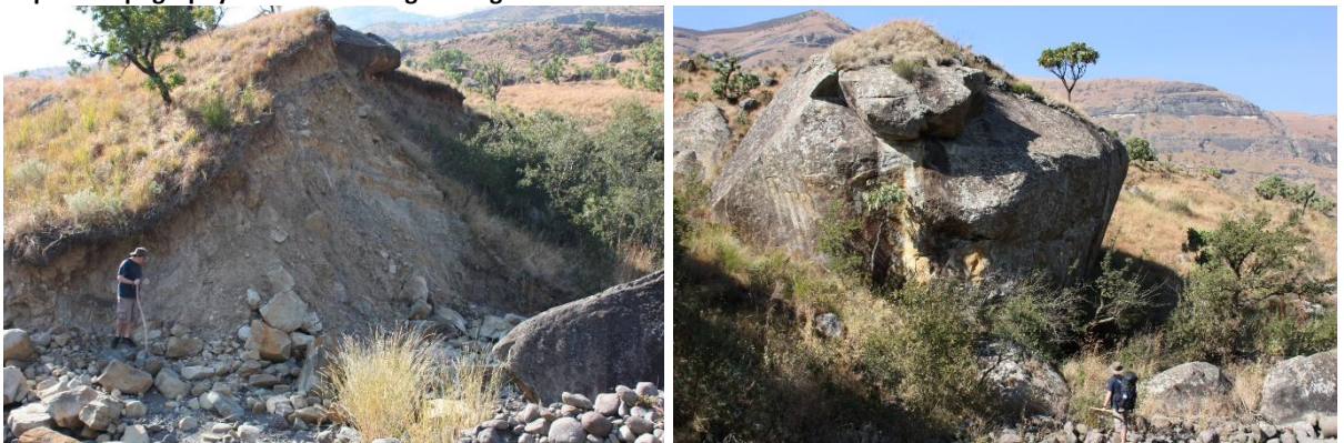
Figure 5.8: (Left) Weathering and erosion of the toe near the left flank exposes angular boulders within the soil which indicate a colluvial disposition. (Right) Massive boulders are located within the regolith on the toe of the movement near the right flank.
