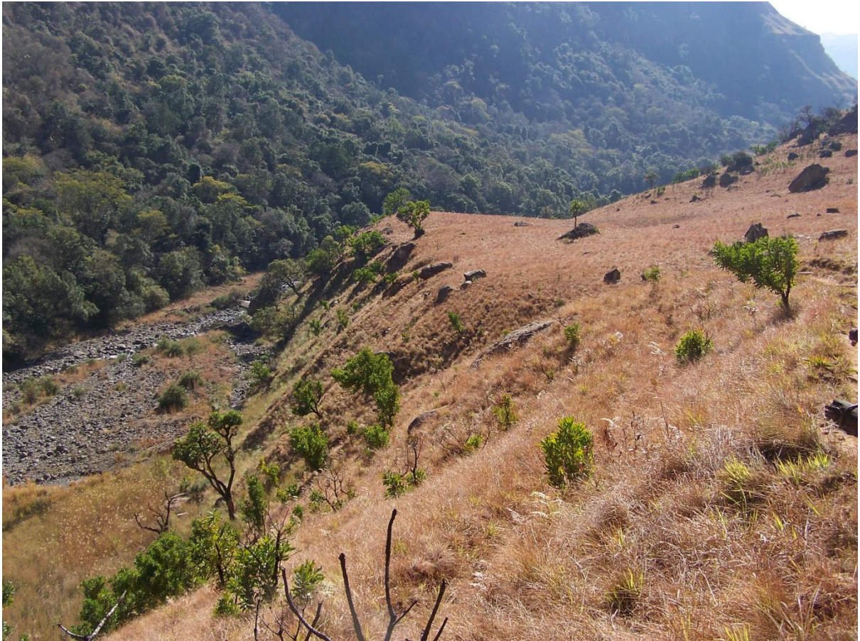
Figure 5.44: View from backscarp towards the left flank and foot of the movement. Clear valley pinching is visible.
