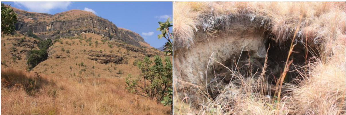
Figure 5.31: (Left) A collapsed soil pipe found on the left flank of the Mushroom Rock movement. (Right) A view from the left edge of the movement towards the back scarp.
