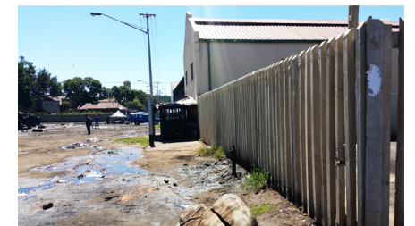
Fig.157. Parking lot and Tamil Hall
