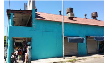
Fig.87. Empire Theatre adaptive reuse.
