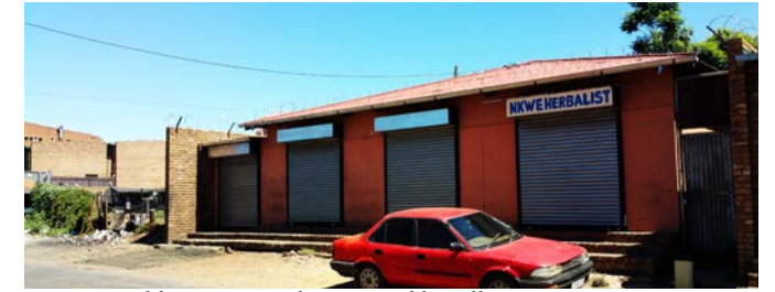
Fig.88. Buildings converted into rentable stalls.
