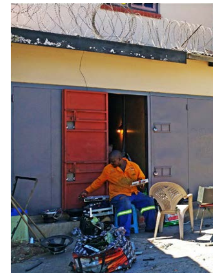
Fig.65. Electrician using the pavement as workshop space.
