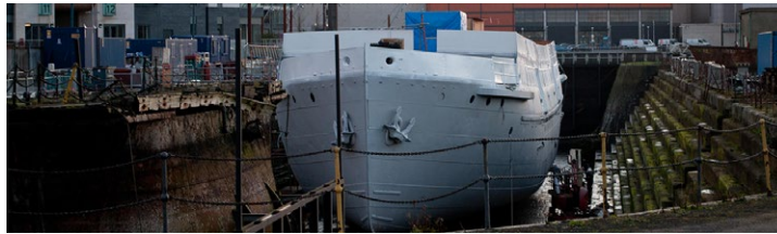
Figure 2.43. Restoration of the SS Nomadic's Hull (Wilson, 2011)
