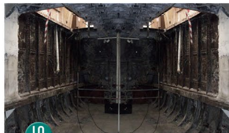
18 empty boiler room fore view
