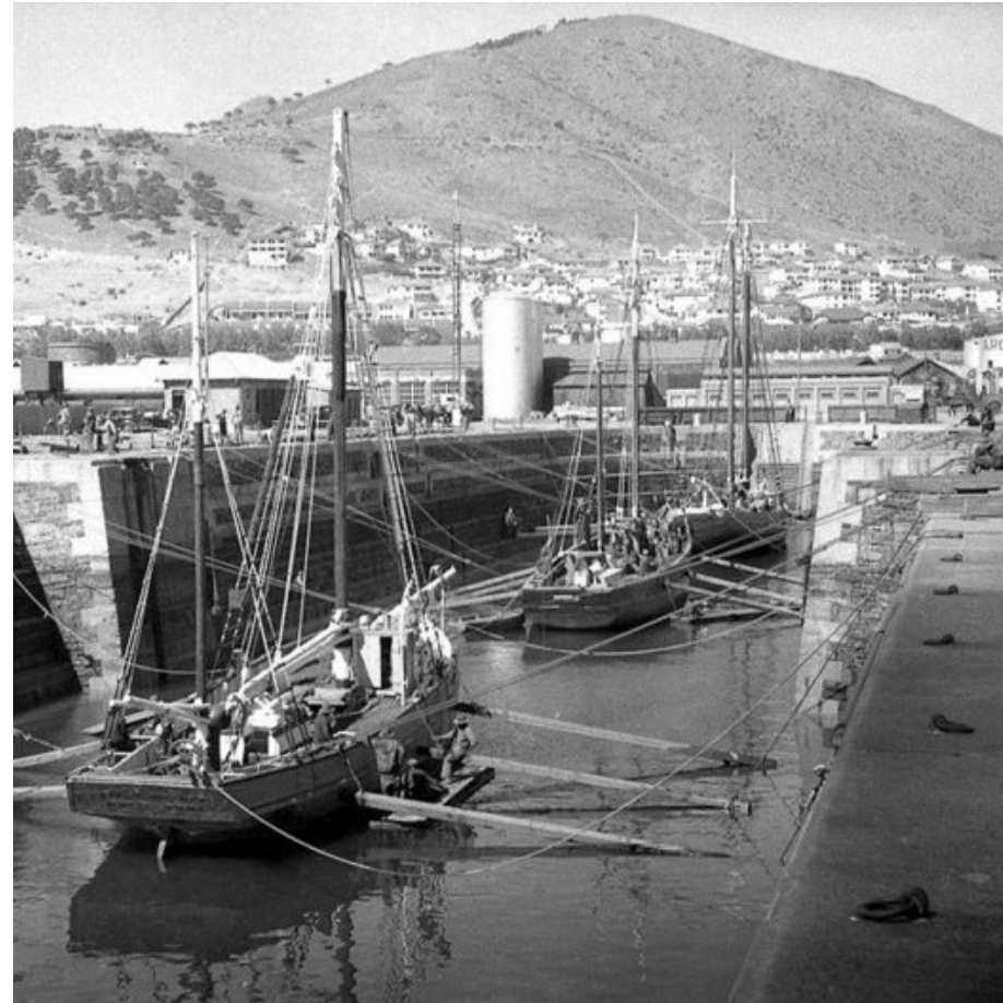
Figure 2.4. Robinson Dry Dock in Service (NPA, 1882)
