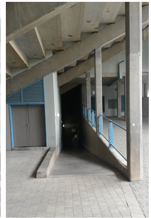
Ramp to basement warm up area
