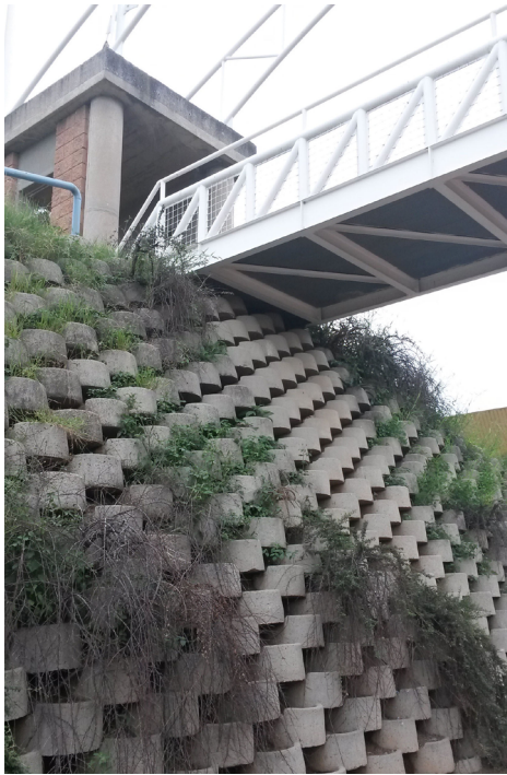
Bridge connecting the berm
