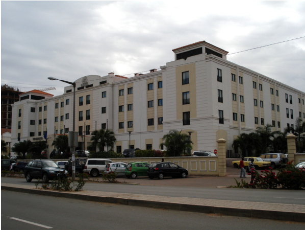
FIGURE 19: New hotel development in expanded city centre.
