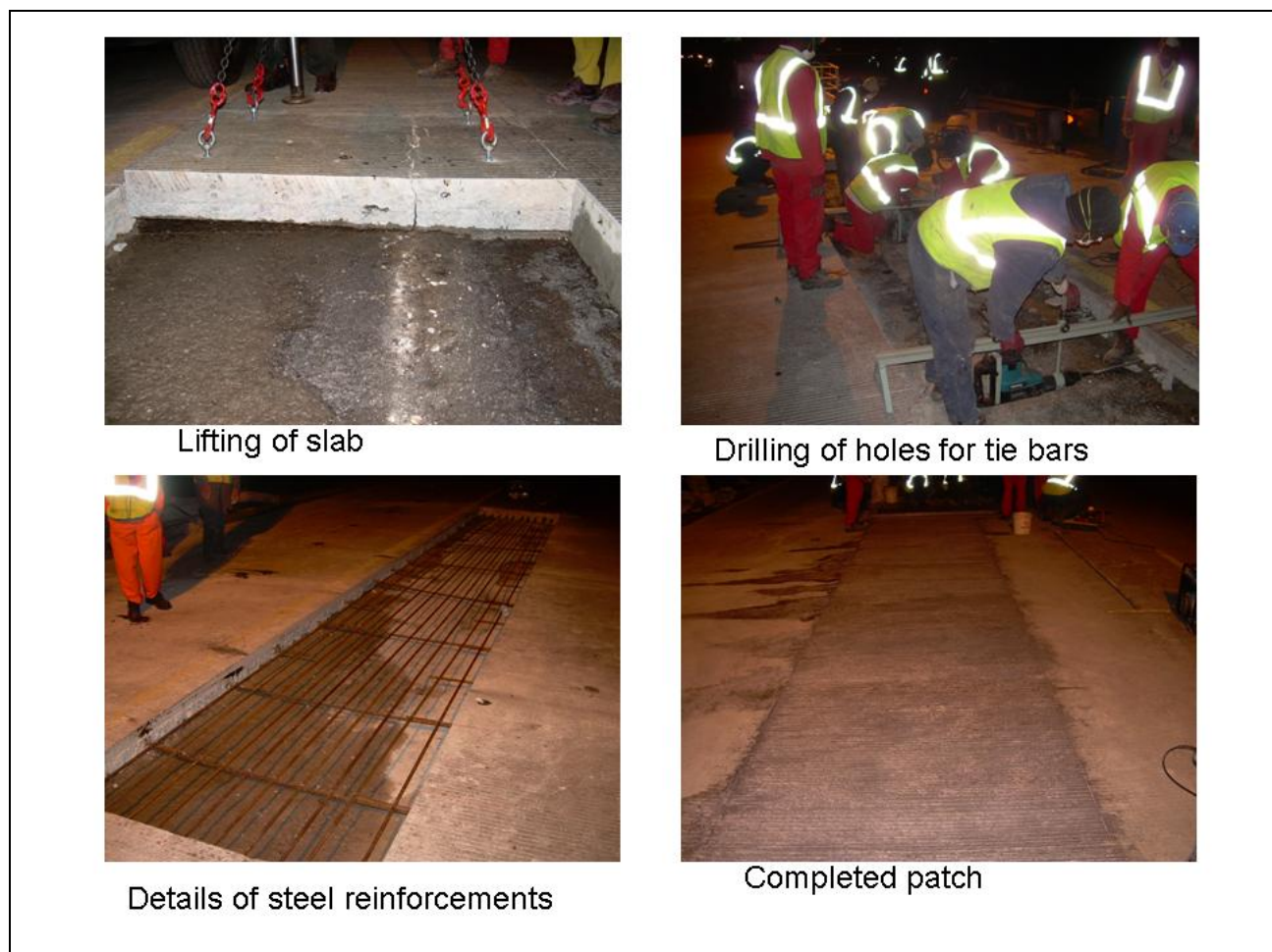
Figure 1: Typical construction activities
