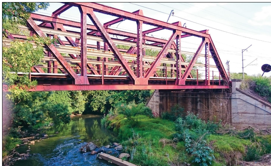
Figure 1 Side view of the bridge
