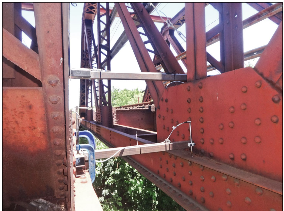
Figure 7 Displacement transducer fixed at point a
