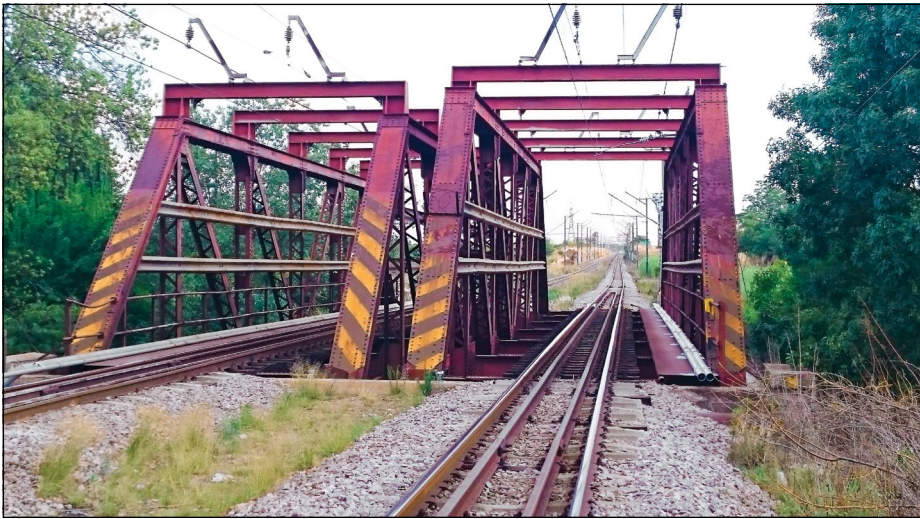
Figure 2 End view of the bridge
