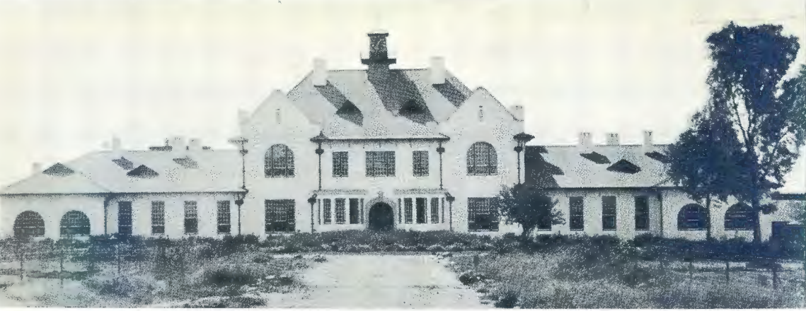
The Main Building at Onderstepoort, 1908.
