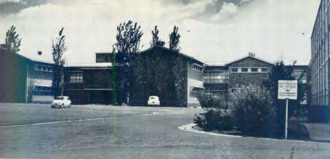
The faculty buildings.
