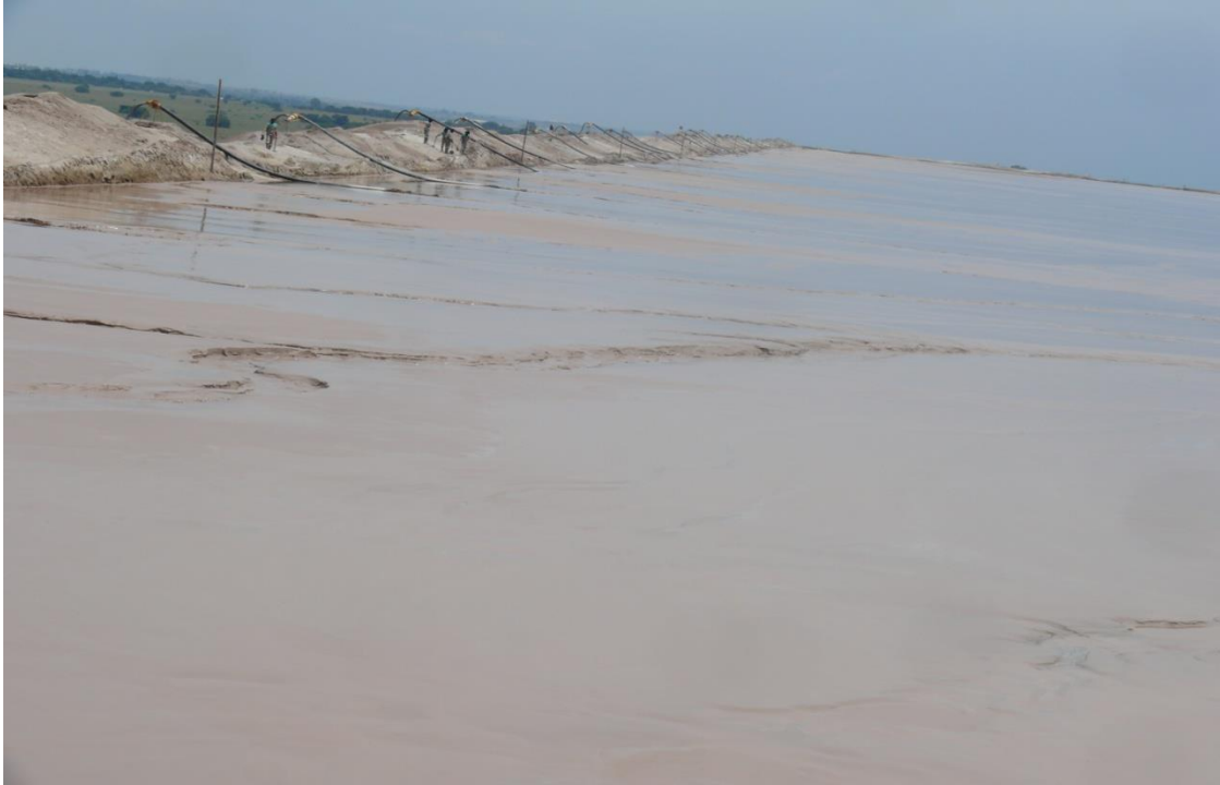
Figure 3.3: Chemwes Dam 5 dam wall and beach area
