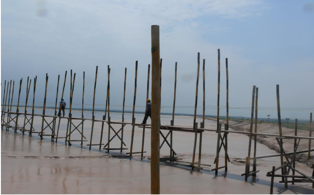
Figure 3.6b: Chemwes Dam 5 the start of catwalk leading to the penstock
