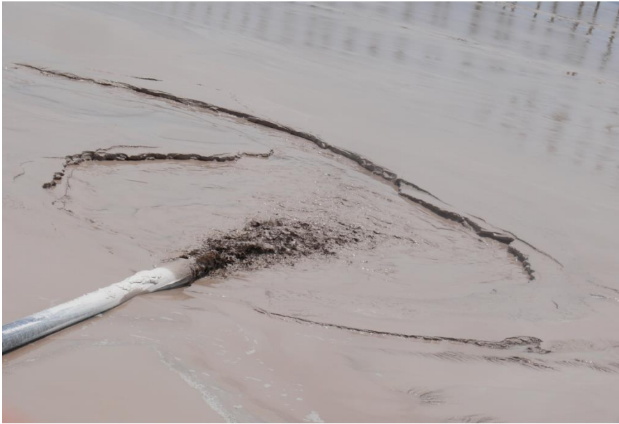
Figure 3.7: Chemwes Dam 5 overflow tailings depositing on the beach area with channelling forming at the discharge point and along the dam beach area.
