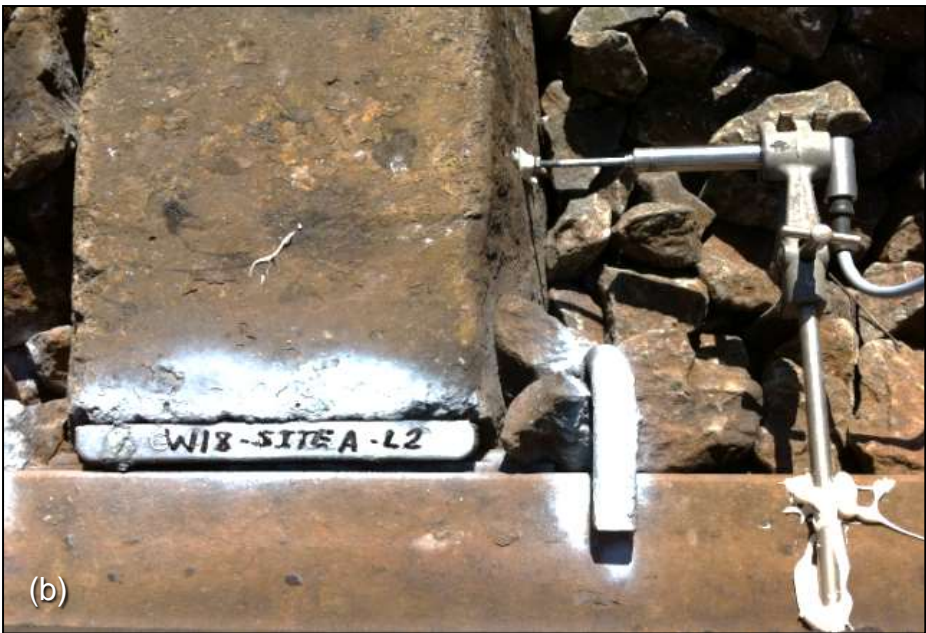
Figure 7. Setup of LVDTs for deflection measurement of the rail relative to the sleeper: (a) Site A with instrumentation at 4 fastenings (b) Site A instrumentation at position L2
