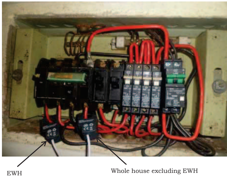
Figure 4.3: Connection at the DB
