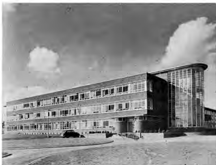
A classroom wing of the Sidcup and Chislehurst School completed in 1938 for the Kent County Council. The school can accommodate 660 boys.
