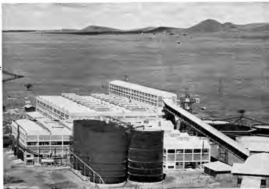
REDUCTION PLANT, LIBANON GOLD MINE
