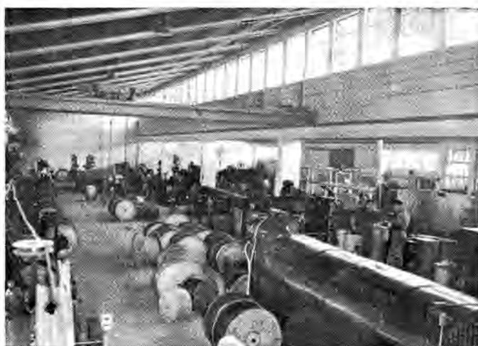
The plastic tuber, laying up and brading machines at the new Asea cable factory, at Pretoria.
