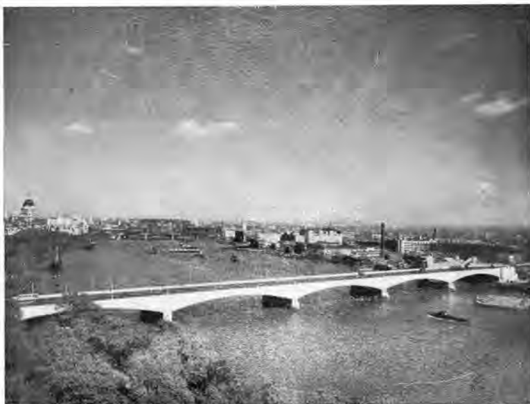
The new Waterloo bridge which takes the place of Rennie's original structure.
