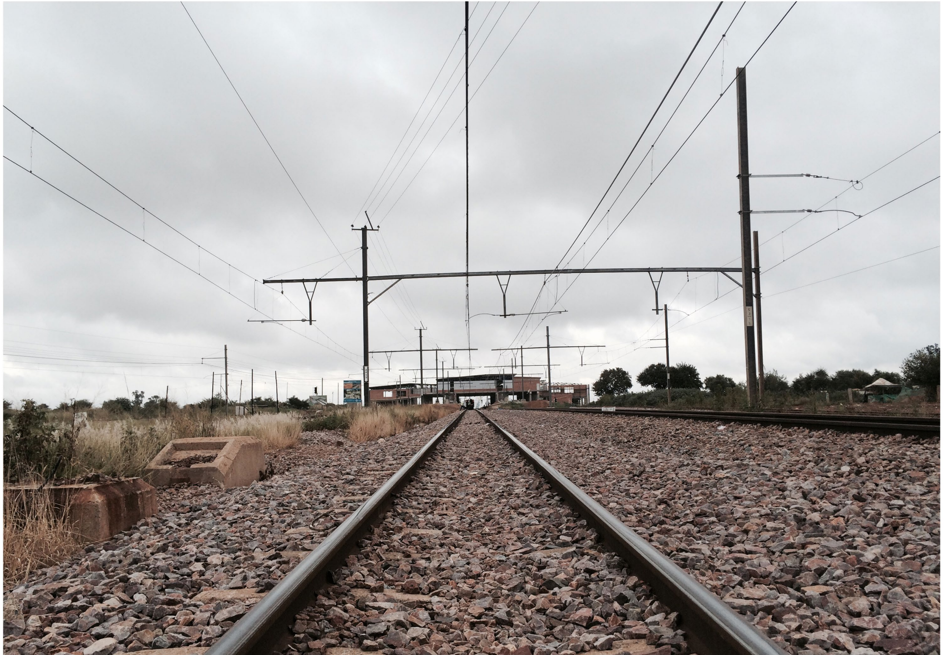
Fig. 1.9 Newly renovated GreenView Station
