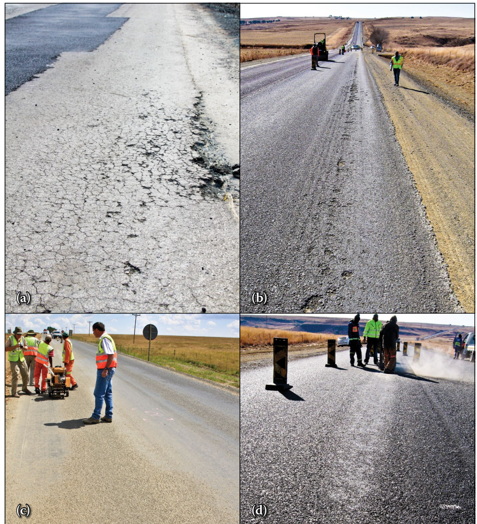
Figure 2 Examples of premature failures at case study sites: (a) general surface failure, (b) rutting and aggregate loss in wheel tracks, (c) bleeding in wheel tracks, (d) bleeding in isolated areas
