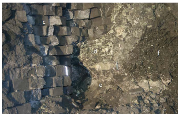
Figure 7 —Detail of tap-hole B with (c) SiC bricks, (d) slag with burden and/or coke bed material, (e) mixed material containing metal, and (f) clay mushroom infiltrated with slag
