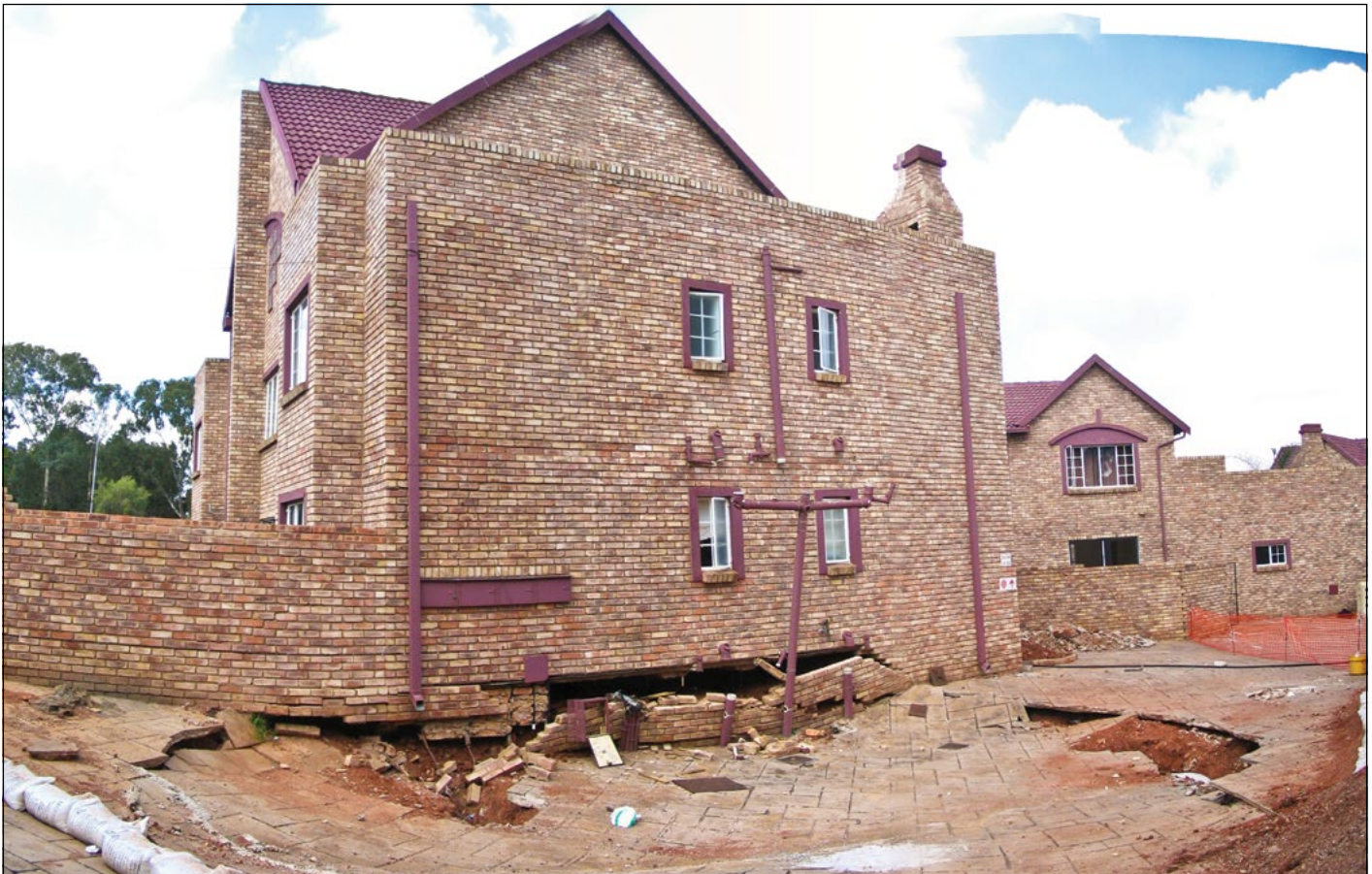
Photo 2 A sinkhole that occurred in a residential complex, which led to the demolition of two units
