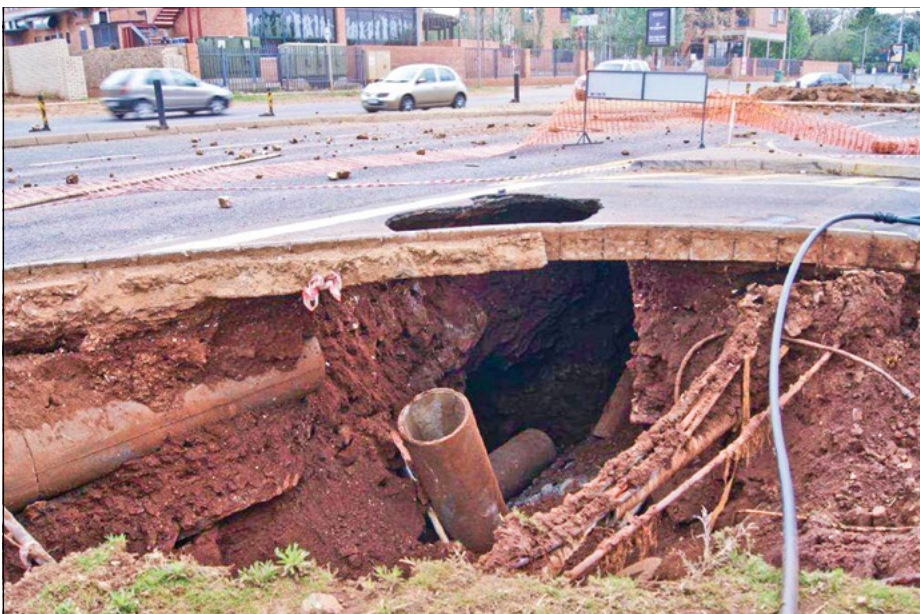
Photo 1 A sinkhole that occurred in Jean Avenue (2012), costing millions of rand to repair
