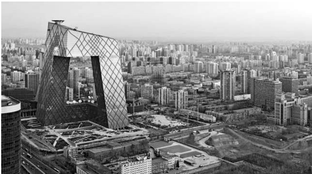
3.8 Rupture through scale CCTV building in Beijing, OMA.
