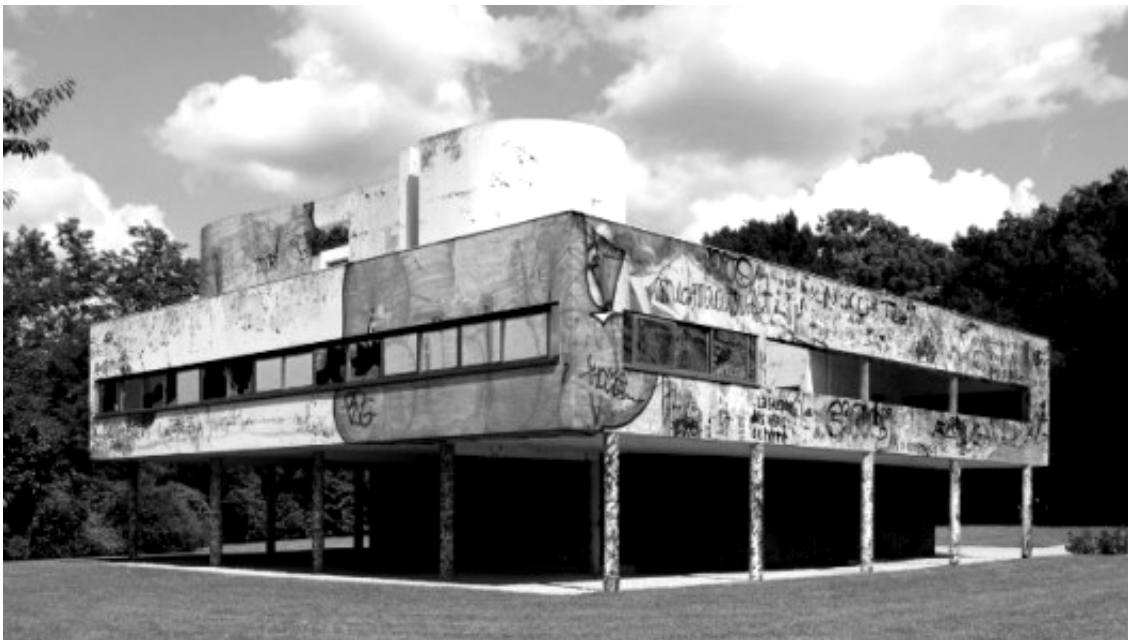
4.9 The pressure of perfection 'Vandalised' Villa Savoy, Xavier Delory
