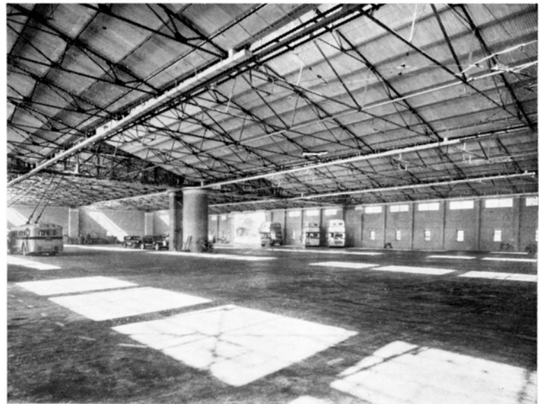
THE PARKING GARAGE: Note the massive, brick-lined central pier supporting the trestle girders. The floor area is 300 ft. x 200 ft.
