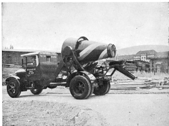
A Continental motor lorry fitted with a rotating drum, used for conveying ready-mixed concrete from factory to building site.
