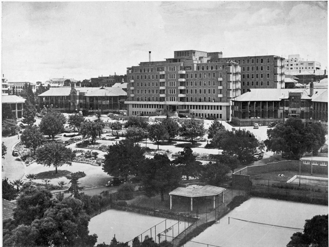
NEW CENTRE BLOCK : GENERAL HOSPITAL : JOHANNESBURG. [Photo S.A.R. & H.]
