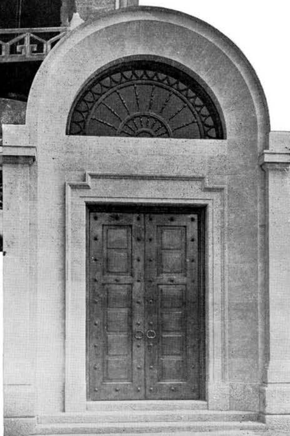
Example of Heavy Plate Bronze Metal Door, with Welded Angles. NEW GOVERNMENT OFFICES, PRETORIA.
