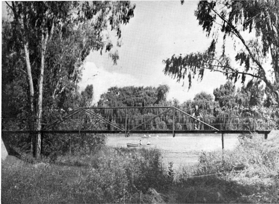
Welded Steel Tubular Bridge at the Country Club Golf Course, Vereeniging Manufactured at our Vereeniging Works.
