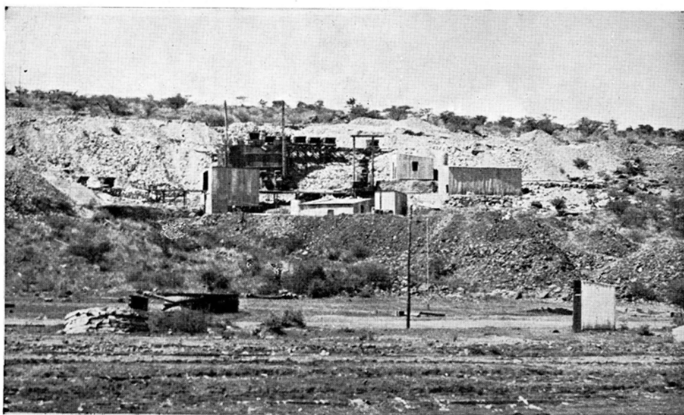
THE VAAL-HARTZ IRRIGATION SCHEME: CRUSHING PLANT AT POKWANI, WHERE THE PRODUCT OF THE TUNNEL WAS CRUSHED FOR CONCRETE AGGREGATE. (Photo: Erik Todd.)
